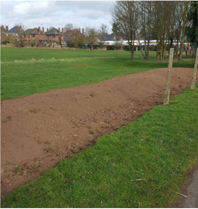
Example ditch and mounding under construction
