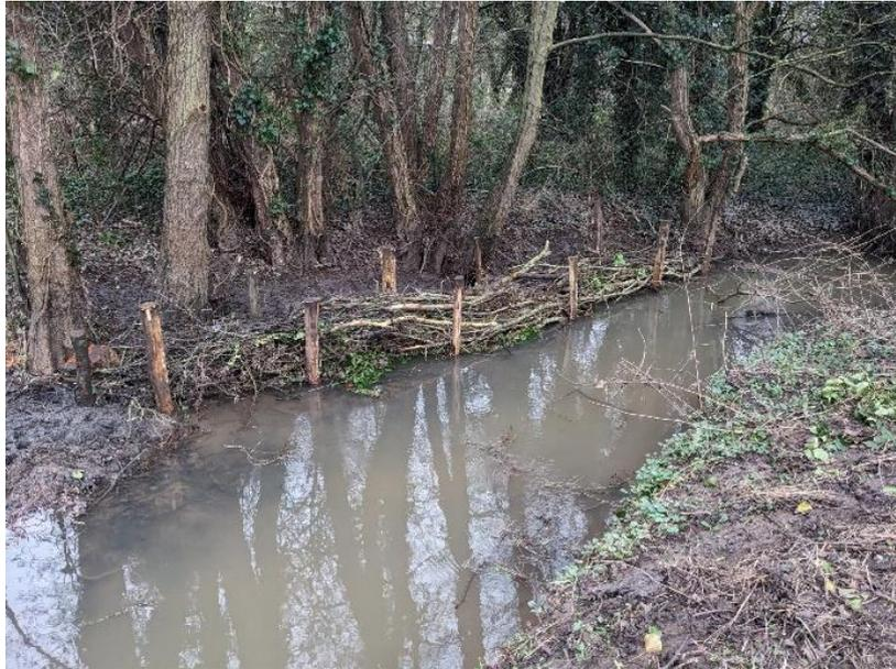
Erosion control areas where woody brush is placed and pinned between the posts (before and after below)
