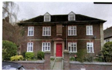
Teacher's House , Church Lane Grade II Listed.
