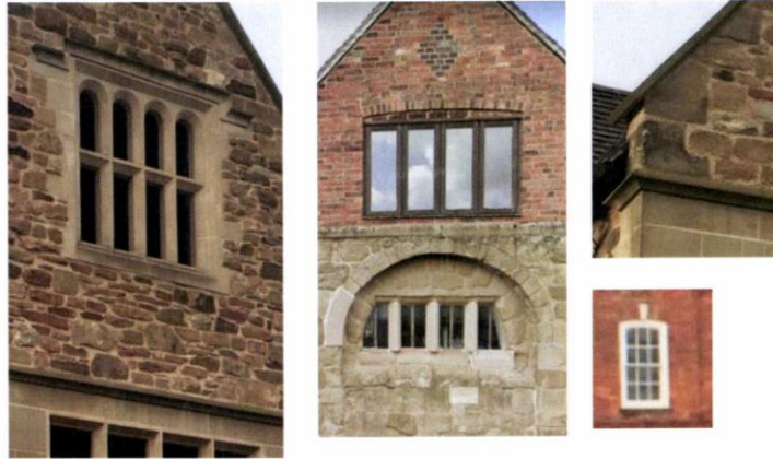
Examples of local characteristics and detailing: common use of string course and change of façade treatment to different storeys, stone mullions, arched window head, brickwork detailing.
