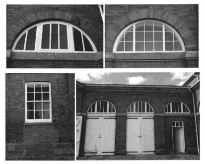
Figure 27: Courtyard windows (clockwise from top left) including mullioned coach house casements, 1970s century multi-paned pivot window, 20<sup>th</sup> century coach house doors and single doorway with fanlight, and bricked up doorway with 19070s sash window
