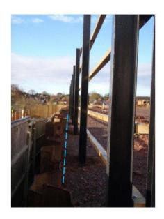
Raised ground level when compared to metal piles and original fence. Paved level will increase height even more.
