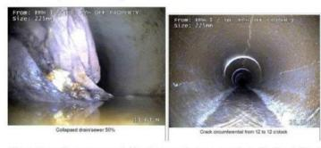
Attached is a professional survey of 40m of sewer under the applicant's site showing significant damage and cracks. Estimated life is 3 years, that's not including all the vibrations from an operational carpark and waste centre above. The high quality materials must now be removed to allow for replacement of entire sewer pipe.
