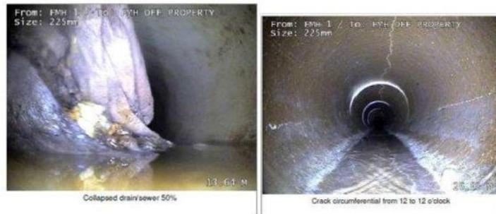
Attached is a professional survey of 40m of sewer under the applicant's site showing significant damage and cracks. Estimated life is 3 years, that's not including all the vibrations from an operational carpark and waste centre above. The high quality materials must now be removed to allow for replacement of entire sewer pipe.
