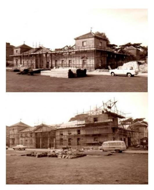
illustrations from 1970 demonstrating the extent of fabric removal undertaken during the refurbishment works
