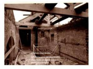
First floor looking north with the bricked up arch to the east elevation visible on the right and the original arch into the counts and on the left.
