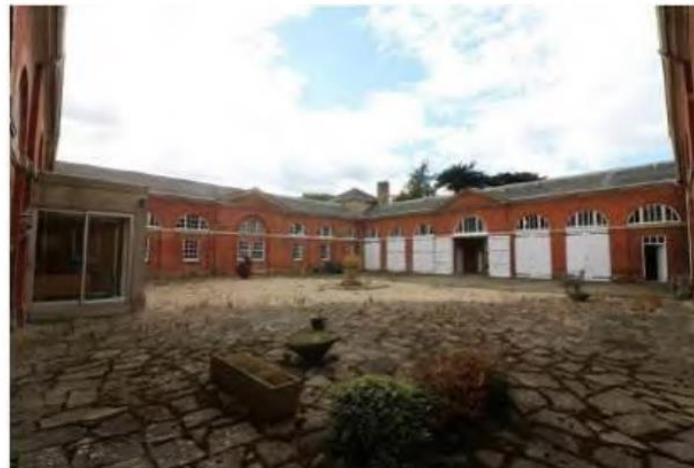
Courtyard north east
