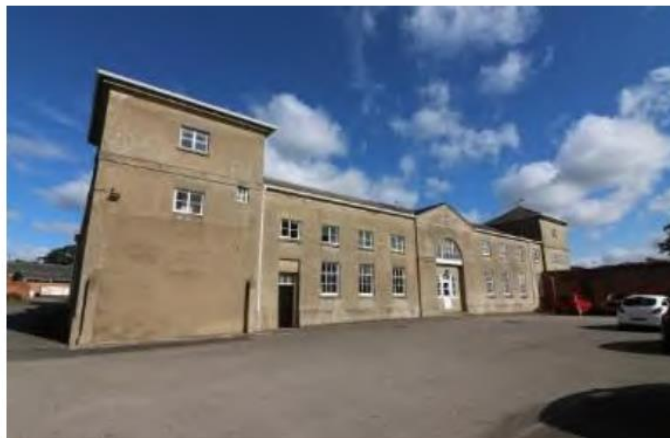
South Elevation – facing north elevation of Hall
