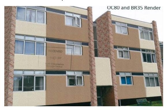
Proposed rear elevation with a contrast light cream and mid brown rendered effect external wall insulation
