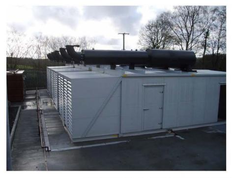
Image of a typical bank of 3 generator canopies (from within an existing compound)
