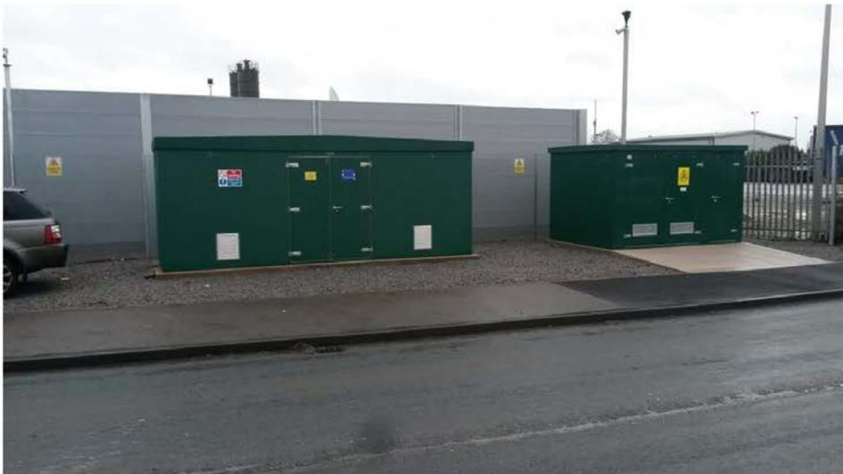
An existing site showing secured compound with internal acoustic fence and external security fence
