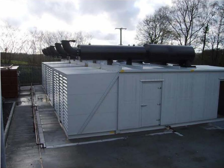
Image of a typical bank of 3 generator canopies (from within an existing compound)
