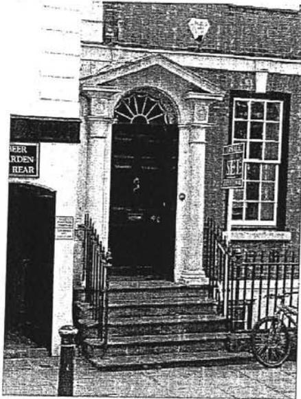
Plate 2. Front steps, railings and doorway with broken pediment
