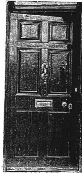
Plate 5. The front door d.1: note the flush flat panels.
