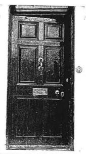
Plate 5. The front door d.1: note the flush flat panels.
