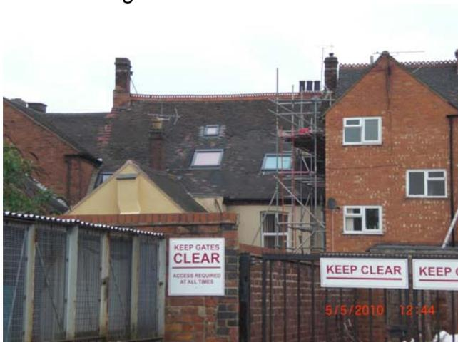
EXAMPLE OF INAPPROPRIATELY LARGE ROOFLIGHTS (REAR OF LONG STREET)
