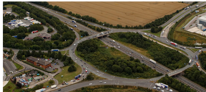
1 Junction 10 M42 Roundabout
