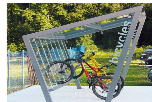
Covered cycle storage
