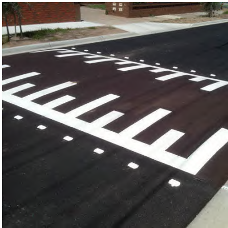
Reflective Road Marking
