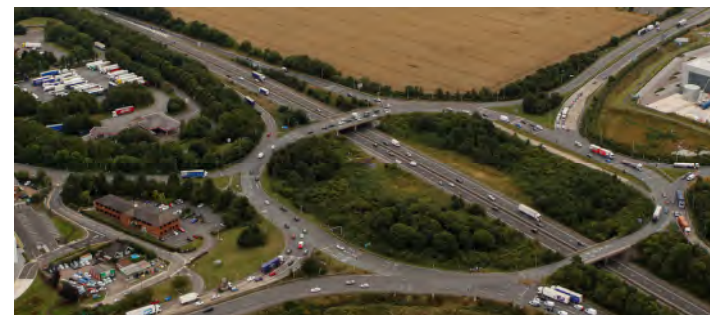
1 Junction 10 M42 Roundabout
