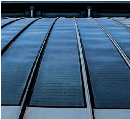
Integrated Solar Panels
