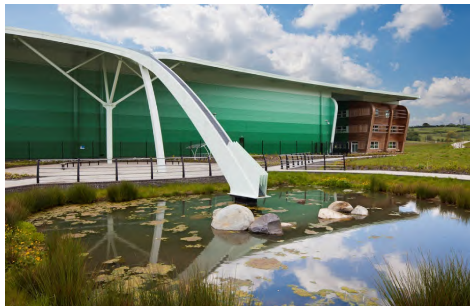
Dynamic roof controls runoff into attenuation pond
