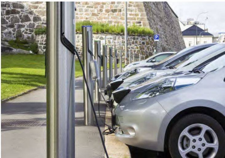
Electric Vehicle charging points
