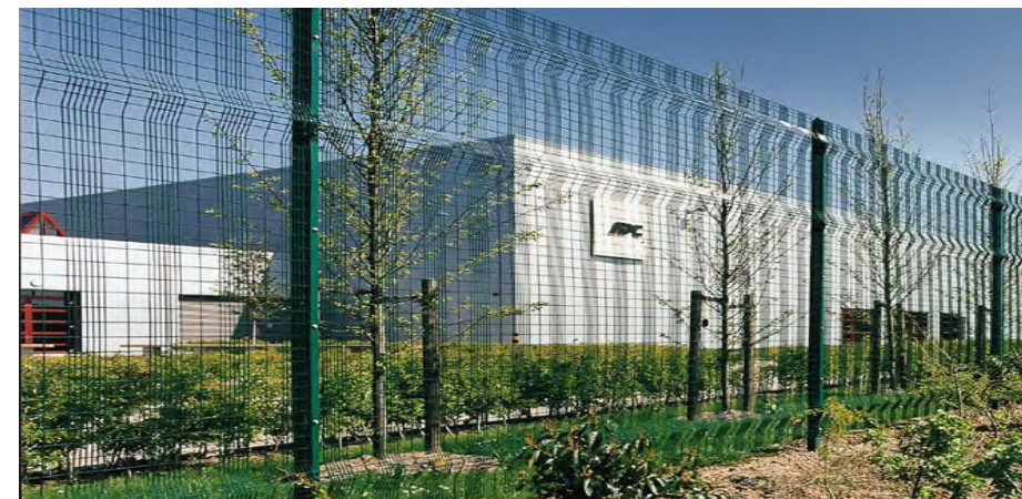
2.4m high palisade fencing
