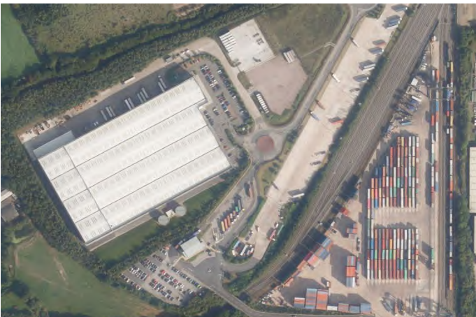
4 Birmingham Intermodal Freight Terminal (BIFT)
