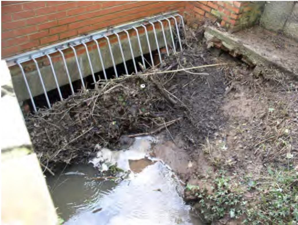
Document 3 – Photograph of Culvert Blocked with Debris
