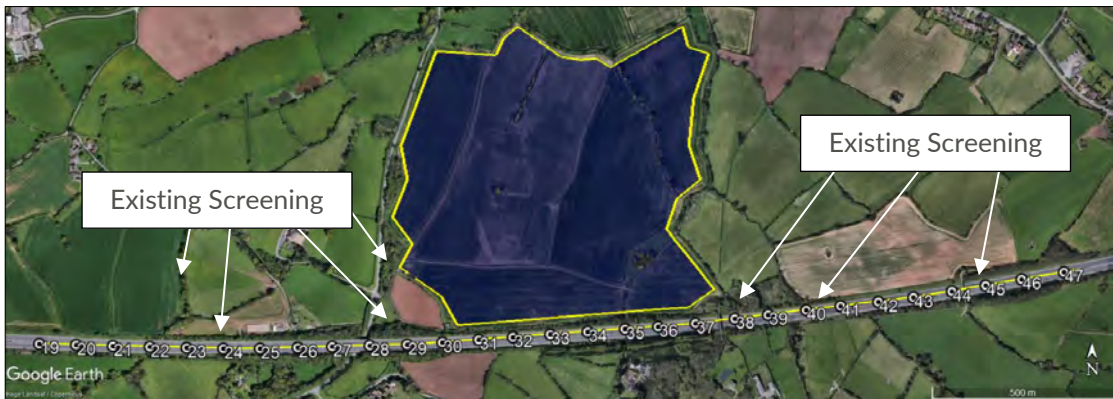
Figure 23 – Stretch of M6 where solar reflections are predicted to be geometrically possible and relevant screening
