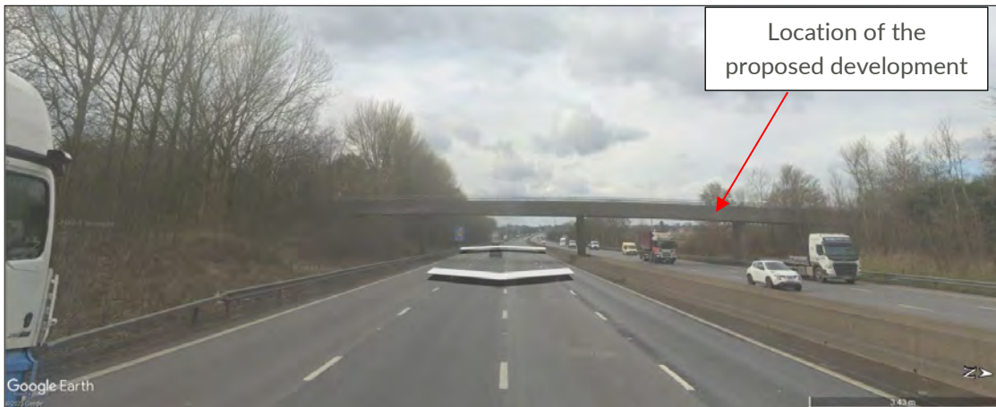
Figure 28 – Level of roadside screening at receptor 38 travelling west (towards receptor 27)
