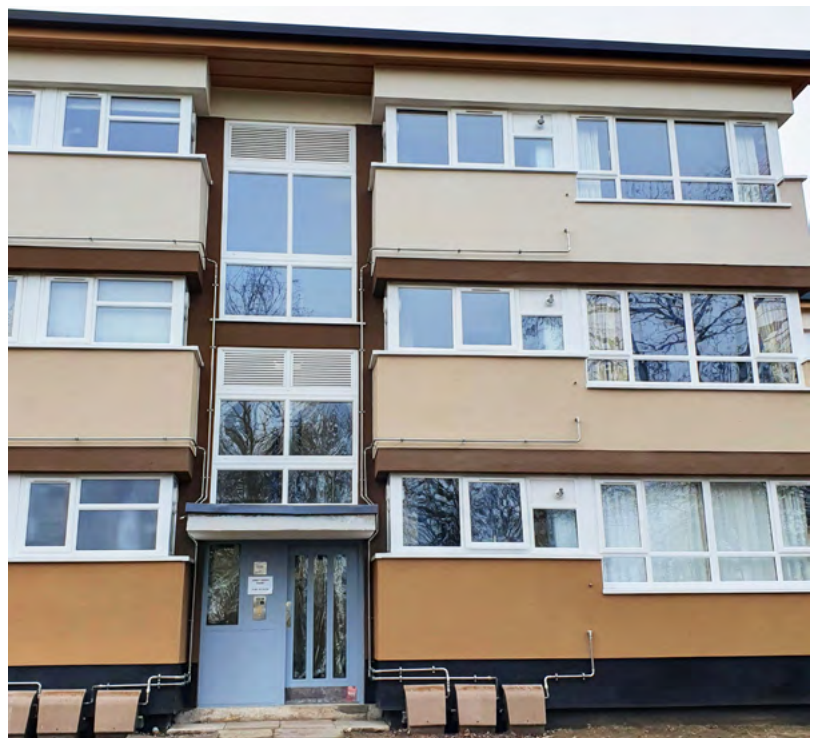
Abbey Green Court following improvement works.
