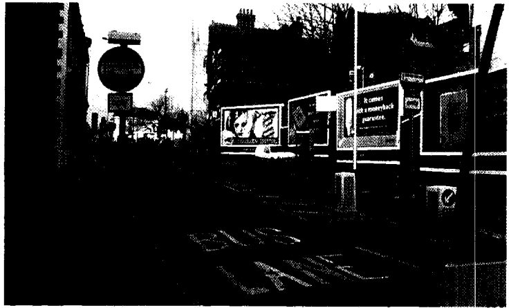
A contra-flow bus lane, separated by islands and road markings.
