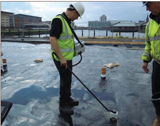
Figure A4.41 Small sand bags are marking holes made in the gas membrane used to check whether injected CO<sub>2</sub> has worked its way beneath whole area (courtesy Landline Ltd)
